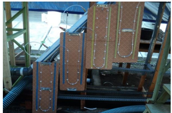
Fig.3 Manometers (with mercury) to observe the pressure change
